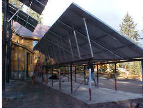
Tilt-up and fixed array mounts on steel or aluminum frames that are set in concrete. This is an example of a well done ground mount.
